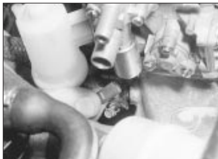
12.7 Disconnecting the float chamber breather solenoid wiring
